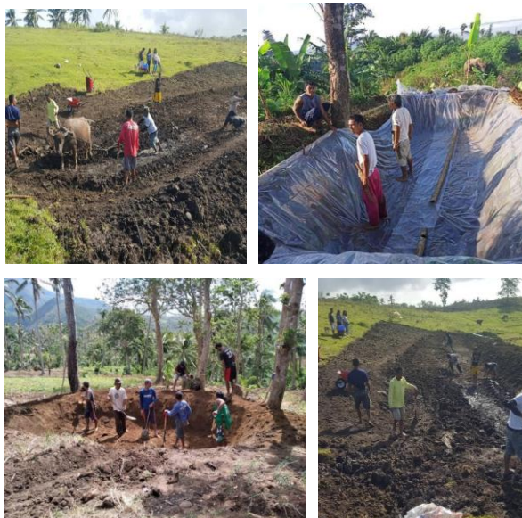
Figure 50: Co-establishment of rainwater harvesting facilities harnessing the collective action (bayanihan) of farmers in the three upland farming communities.
